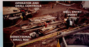
Well drilling procedure
